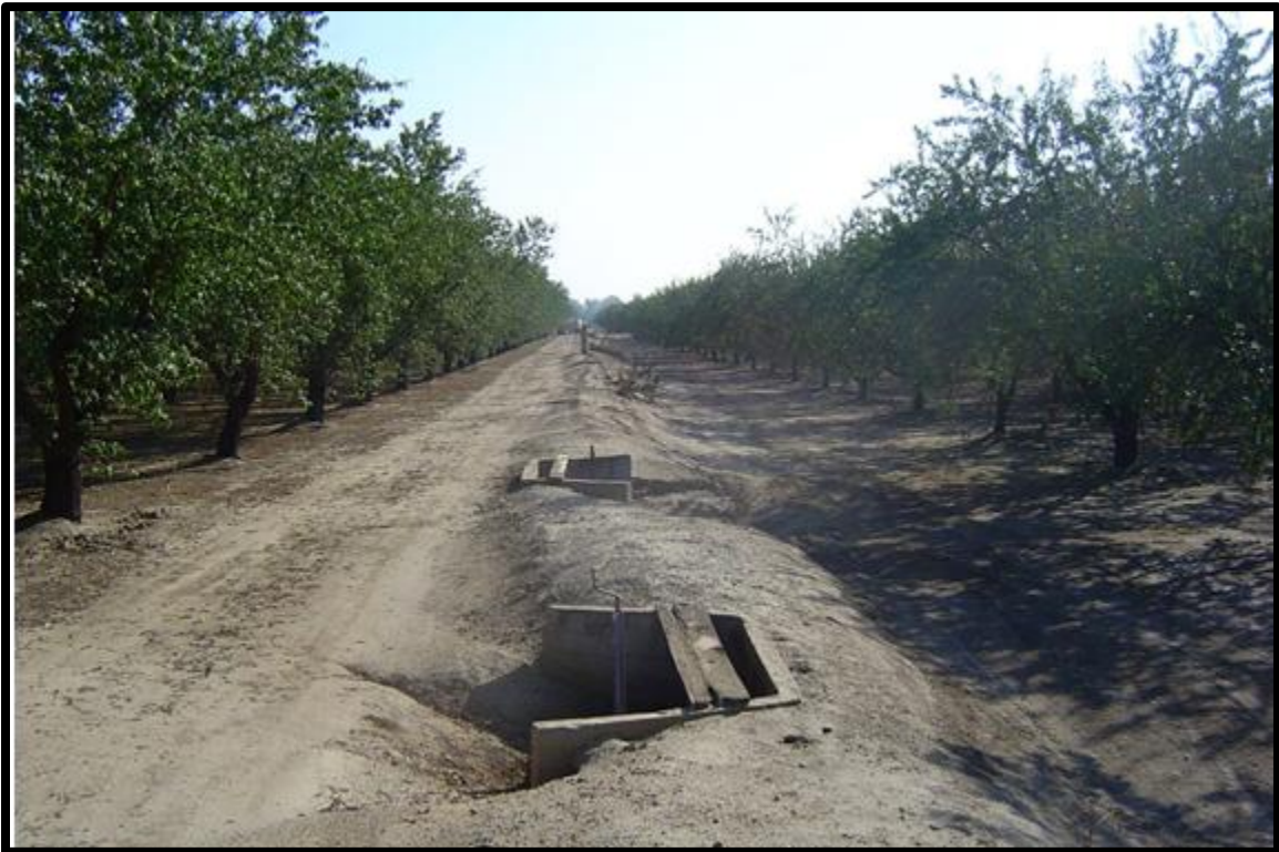
Figure A-3. Multiple valve turnout on a District pipeline.
