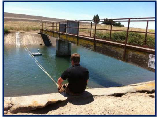
Figure 3-15. Woodward Release Gaging Station
