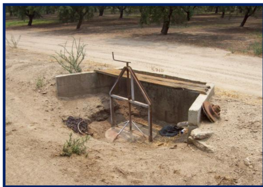
Figure 3-17. Orchard Valve Installed on SSJID Pipeline
