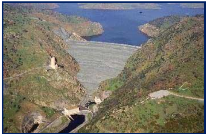
Figure 1-1. New Melones Dam
