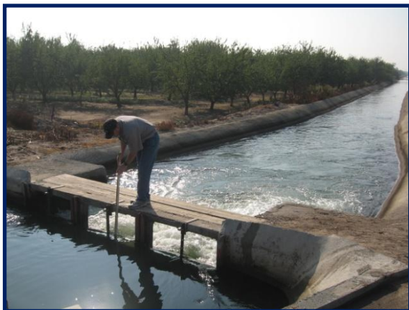
Figure 3-14. SSJID Division Manager Measuring Flow
