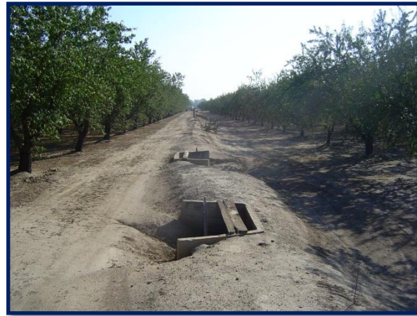
Figure 3-10. Surface Irrigation Valves
