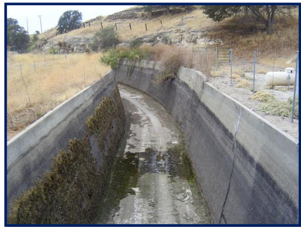
Figure 3-4. SSJID Upper Main Supply Canal
