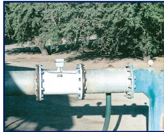
Figure 3-16. Magnetic Flow Meter
