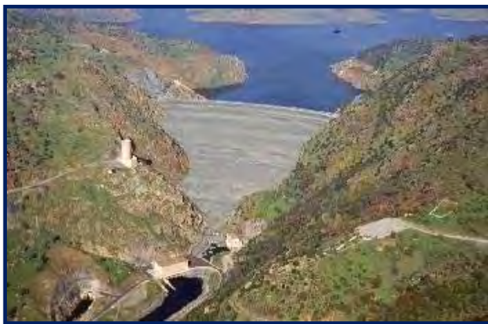
Figure 1-1. New Melones Dam
