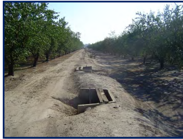
Figure 3-10. Surface Irrigation Valves
