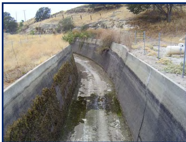
Figure 3-4. SSJID Upper Main Supply Canal
