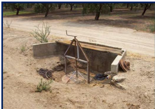
*Figure 3-17. Orchard Valve Installed on SSJID Pipeline*
