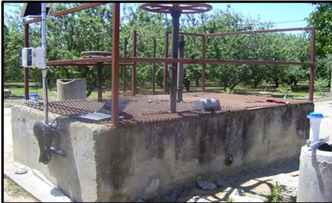
**Figure A-4. Orifice gate turnout in a concrete box on a District pipeline.**
