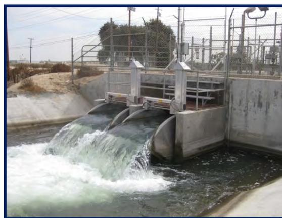
*Figure 3-6. Flume Gates at Lateral Heading*
