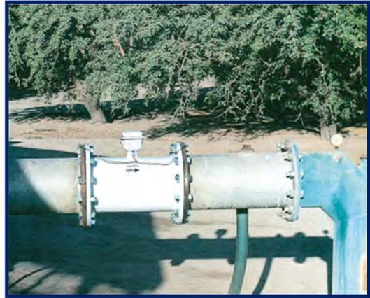
*Figure 3-16. Magnetic Flow Meter*
