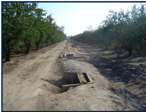
*Figure 3-10. Surface Irrigation Valves*
